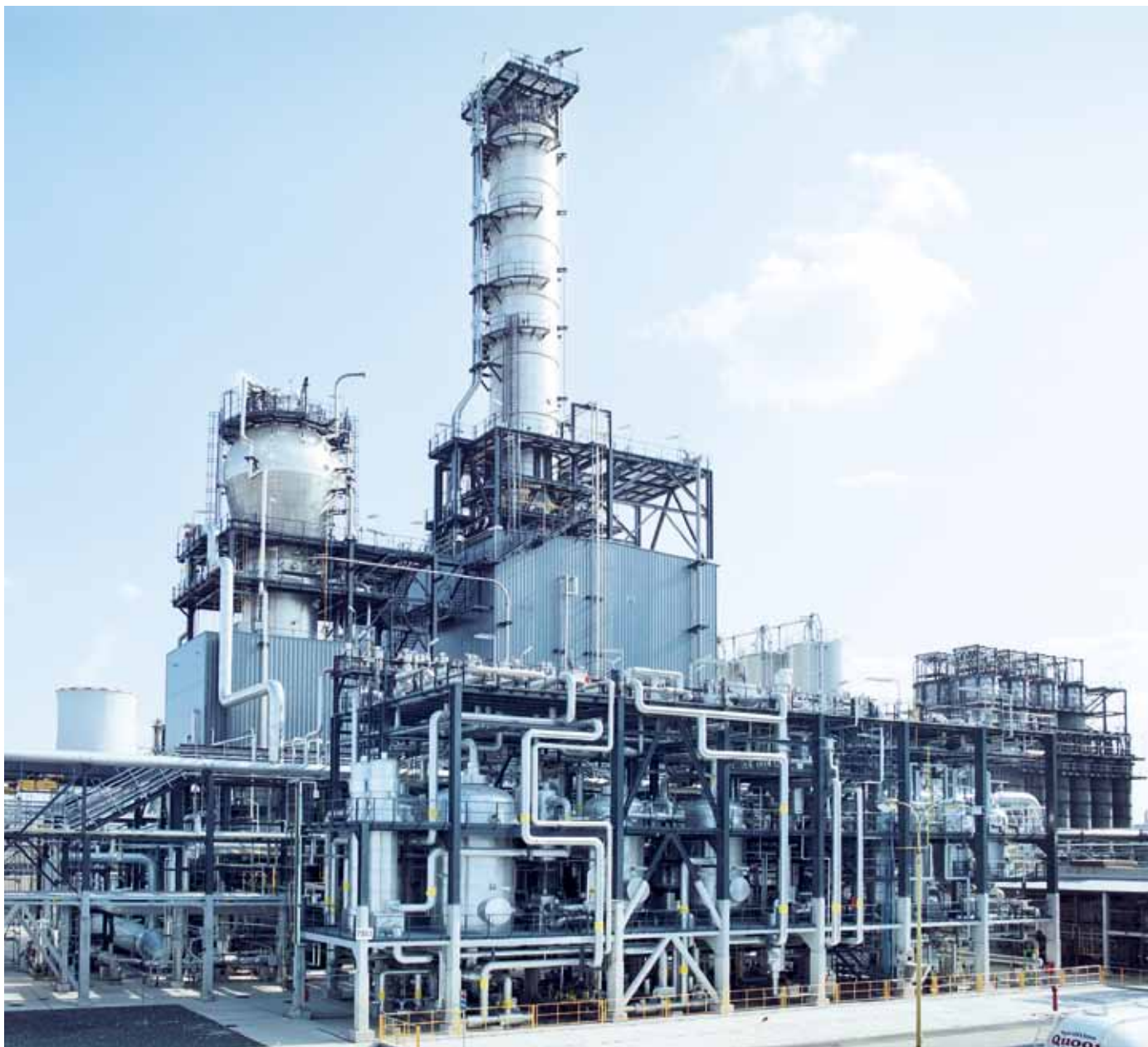
Polyethylenanlage in Litvinov
