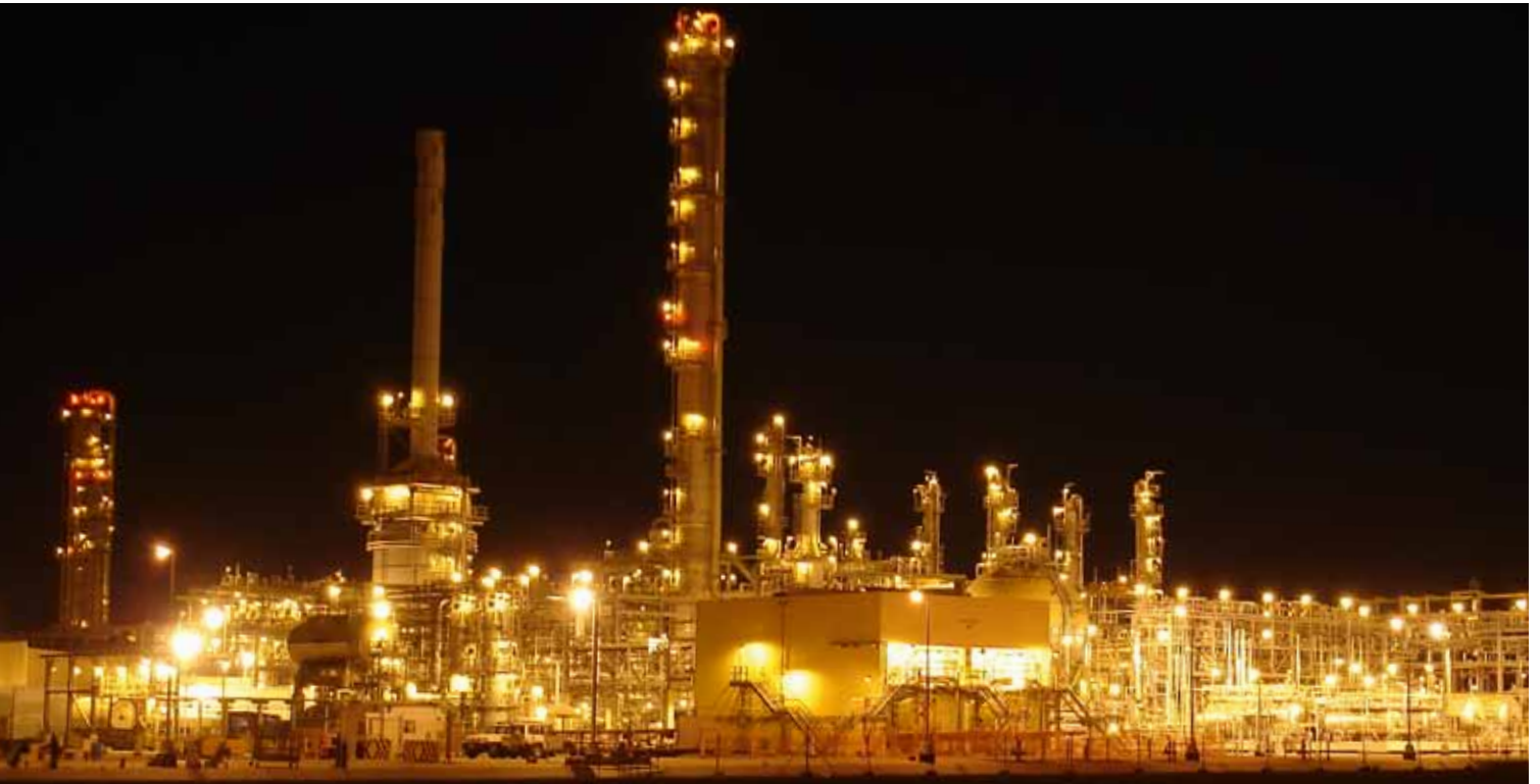
LAO plant in Al-Jubail
